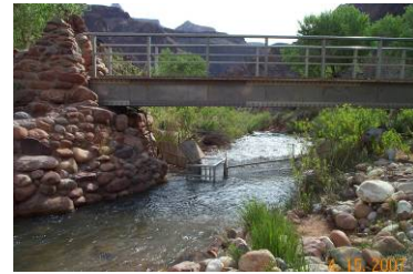
Weir installed in Bright Angel Creek
